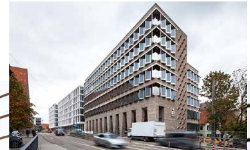
The facade consists of reused bricks.
