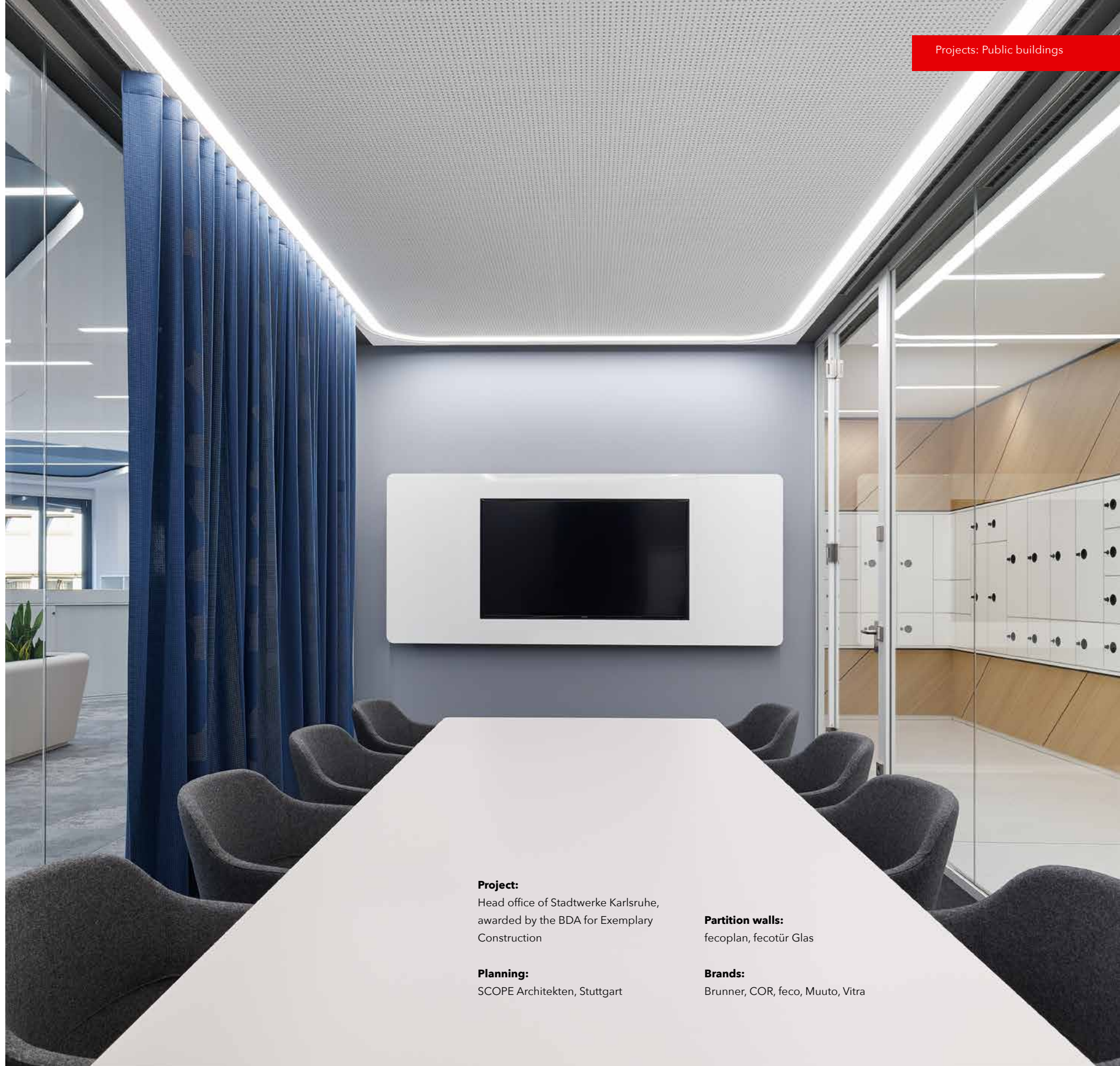
Walls in the fecoplan all-glass construction with all-glass doors with frame-integrated technical door side panels.
