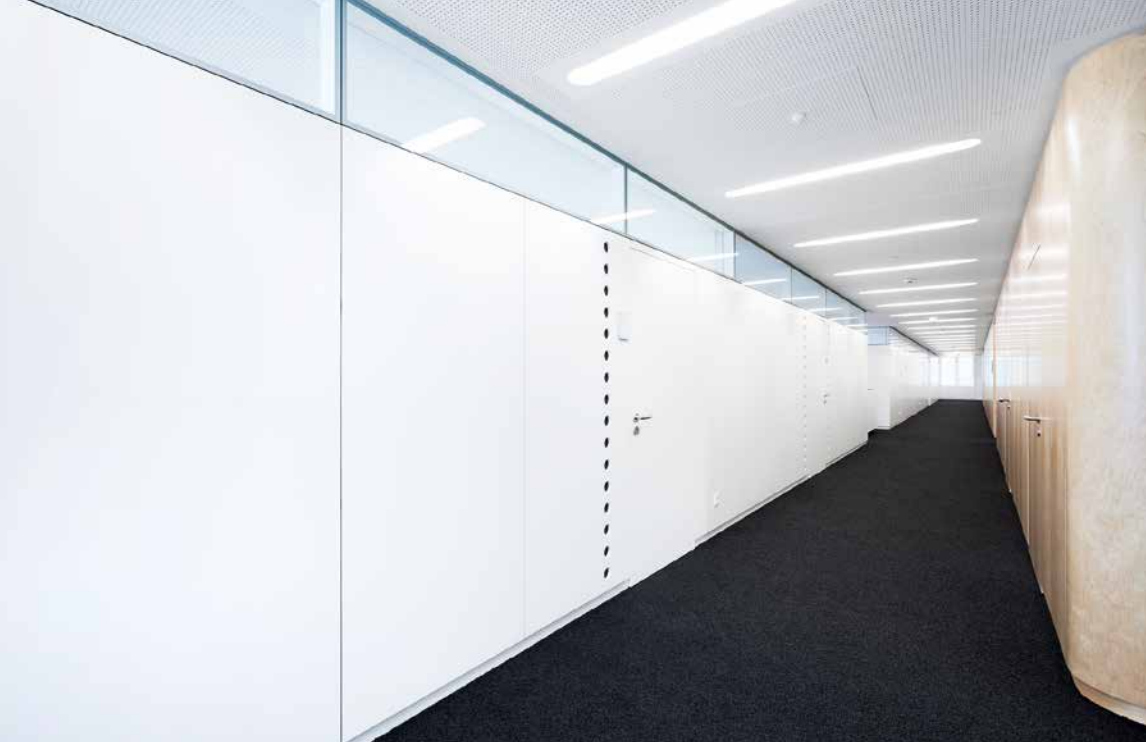
The glass ribbon visually separates the non-load-bearing office partition walls from the concrete-core tempered reinforced ceiling.
