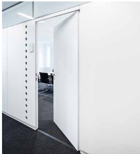
The air is conducted between the offices and corridors with the wall-integrated fecoair overflow elements.
